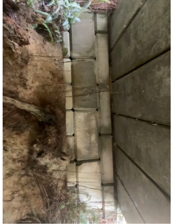
Left Bank Abutment when facing downstream
